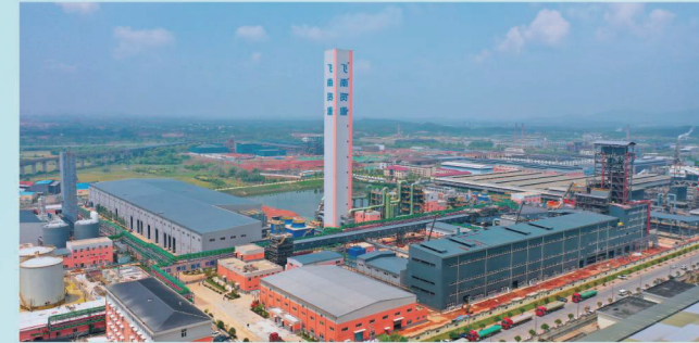
江西兴南危固废处置项目 Project of Hazardous Solid Waste Treatment for Jiangxi Xingnan Environmental Protection Technology Co., Ltd.
