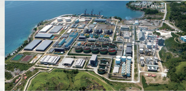
巴布亚新几内亚瑞木镍钴项目 Ramu Nickel-Cobalt Mining, Beneficiation and Smelting Complex, Papua New Guinea
