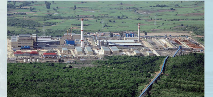
缅甸达贡山镍采选冶联合项目 Tagaung Taung Nickel Mining, Beneficiation and Smelting Complex, Myanmar
