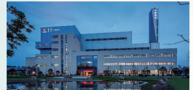
赣州市生活垃圾焚烧发电厂 Project of Domestic Waste Incineration Power Plant in Ganzhou City
