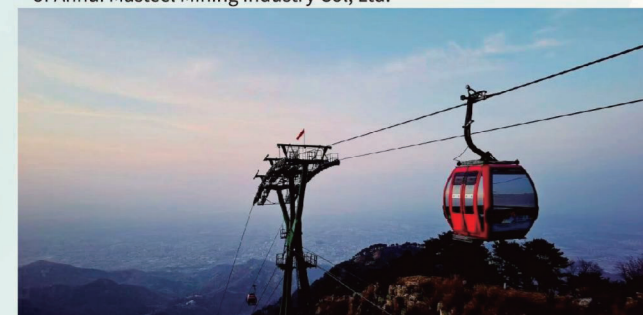
山东泰山中天门索道 Project of Zhongtianmen Ropeway on Mount Tai in Shandong Province
