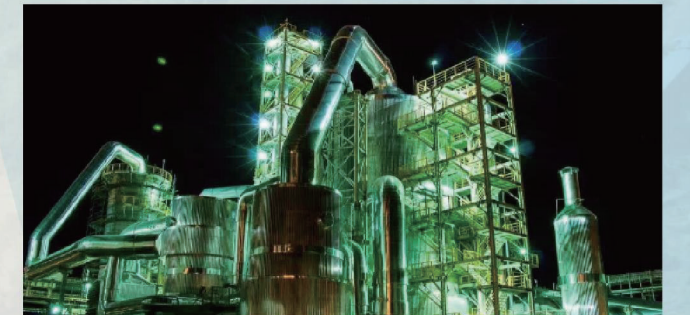
纳米比亚HUSAB 1500 MTP硫磺制酸项目 1500 MTPD SULPHURIC ACID PLANT OF HUSAB MINE IN NAMIBIA
