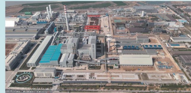
铜陵有色绿色智能铜基新材料项目 Green Intelligent Copper-based New Materials Project of Tongling Nonferrous Metals Group
