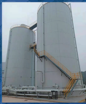
厌氧反应器 Picture 2 Anaerobic reactor
