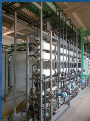
膜处理系统 Picture 1 Membrane treatment system
